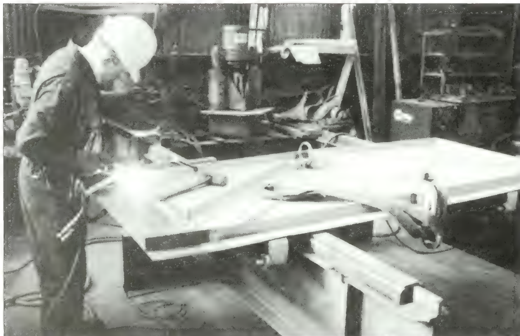
Figure 5.16. Off-site repair of historic metal door for Battery Worth, Fort Casey, Washington. Standing water resulted in the bottom portion of this door being severely deteriorated. The door was removed and is shown being repaired with a new steel plate and angles (From, David M. Hansen, Kimberly Keagle, and Deborah Rehn, Historic Fortification Preservation Handbook , Olympia, WA: Washington State Parks and Recreation Commission, 2003, 3.102).
